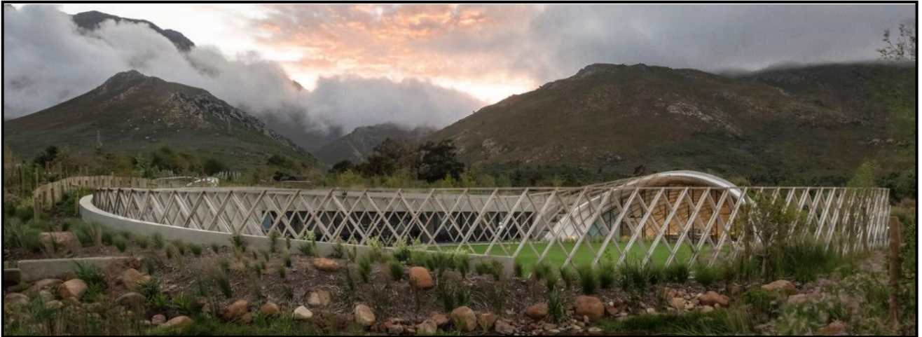
FIGURE 8a: Steyn Studio, Garden Café , curved oak beams, glass and concrete, 2020.
